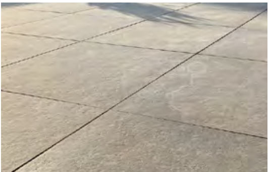
C.I.P. Concrete Paving
