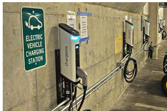
Image 2: Fully Installed Charging Station Sample (EVSE)
